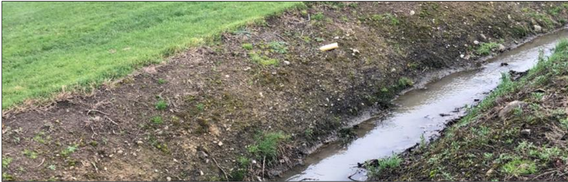
Figure 3: Existing Golf Course Drain
